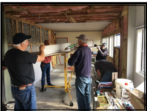
Lining of meeting room with insulation and wall board
